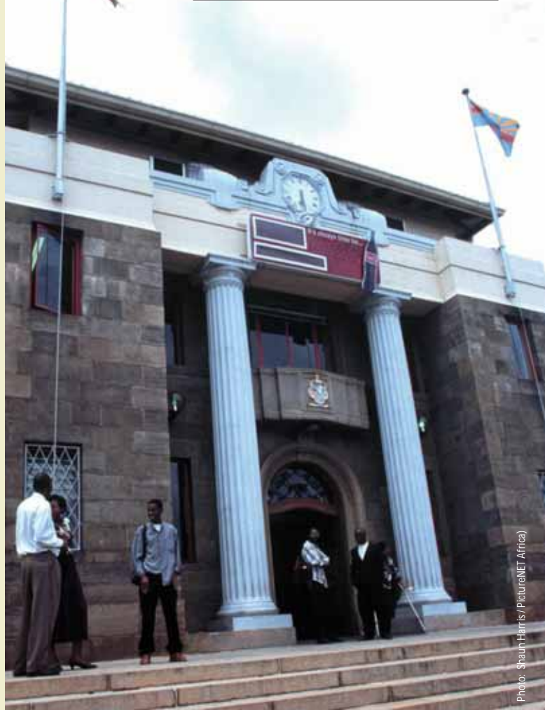
'City House,' the office of the Mayor of Harare in the CBD of Harare, Zimbabwe
